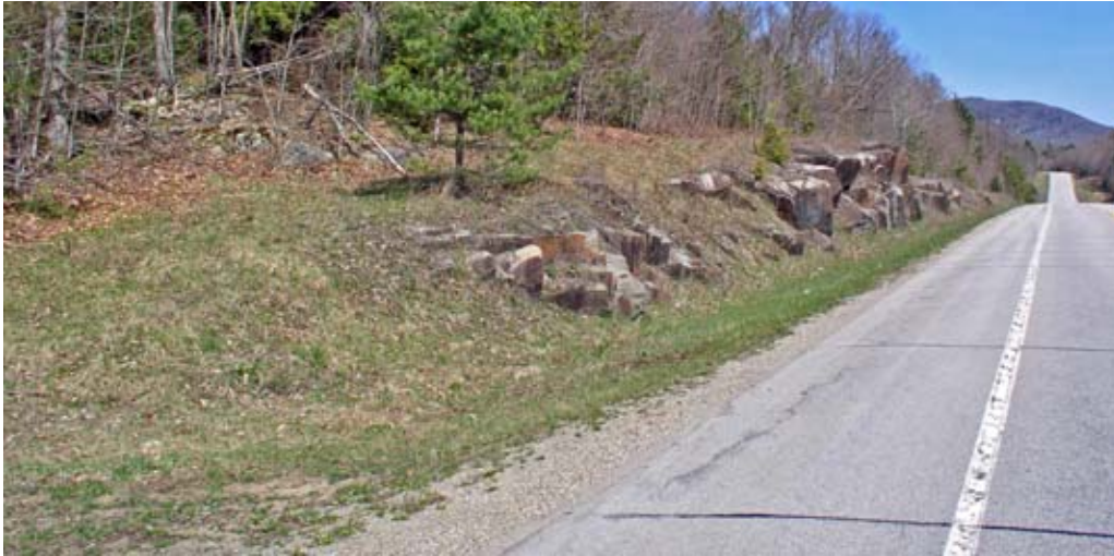
Figure 14.—A highway cut in an area of the Tunbridge-Lyman complex, 15 to 35 percent, very rocky. Scattered areas of rock outcrops make up about 2 to 10 percent of most areas of this unit. Much of the landscape of Hamilton County has massive rock outcrops.
