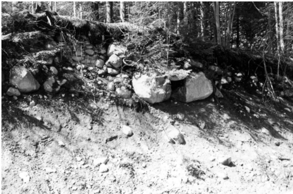
Figure 15.—Roadcut exposing the profile of Monadnock fine sandy loam. Although rock fragments make up as much as 45 percent of the substratum of Monadnock soils, these soils generally are less gravelly and more loamy than associated areas of Colton soils.
